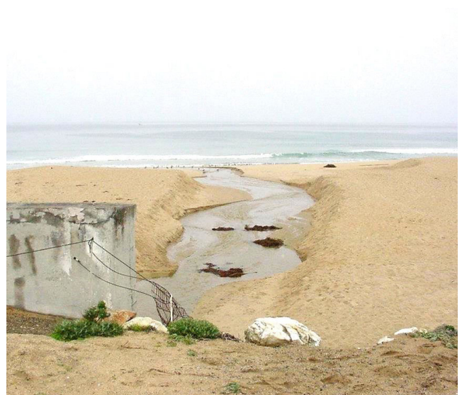
Stormwater Outfall in Seaside.
