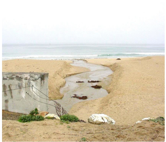
Stormwater Outfall in Seaside.
