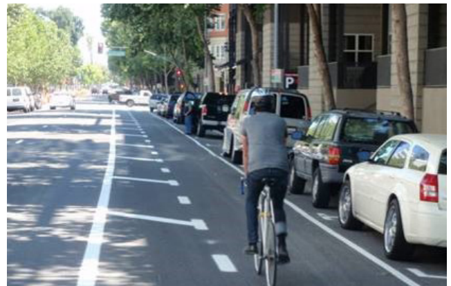
Example of a multimodal street with buffered bicycle lanes.
